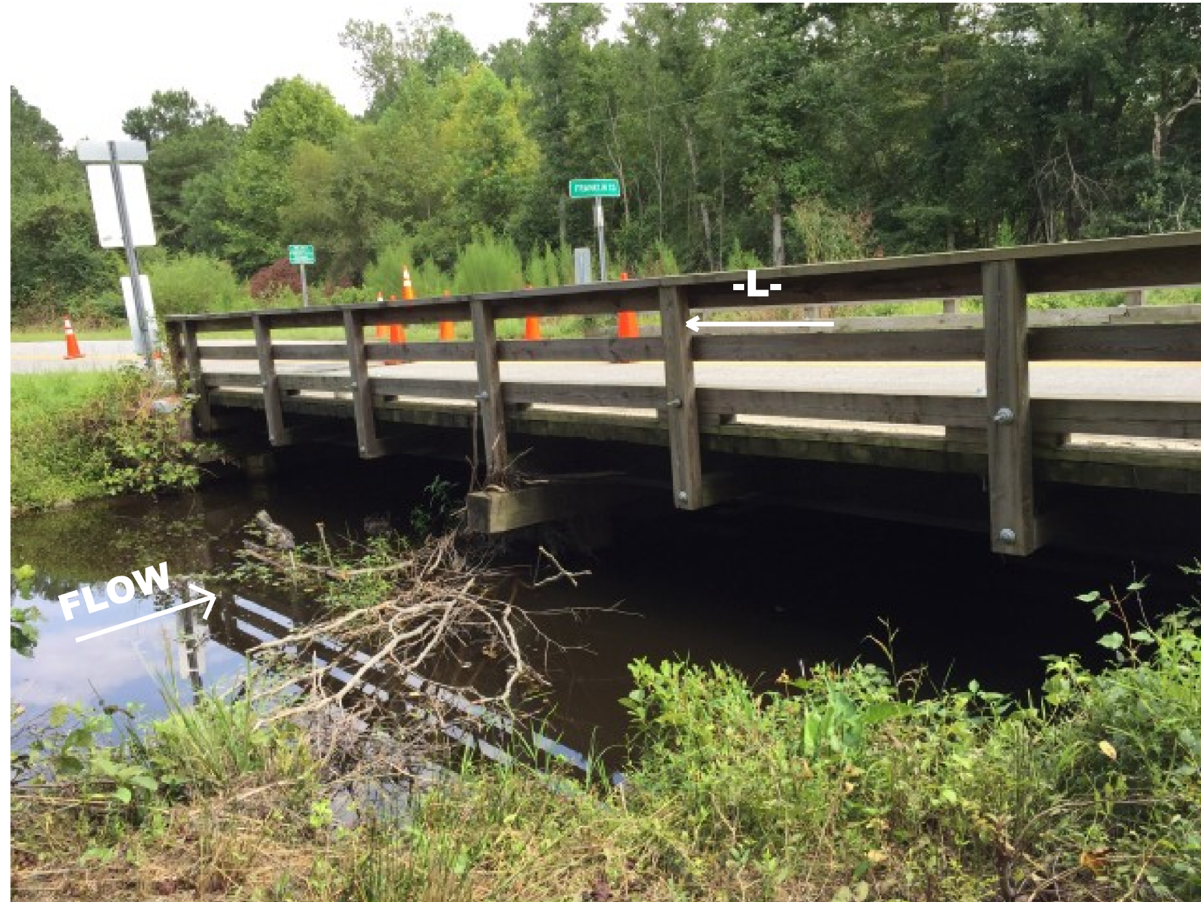
PHOTOGRAPH NO.1. VIEW LOOKING EAST FROM END BENT #1 SIDE.
